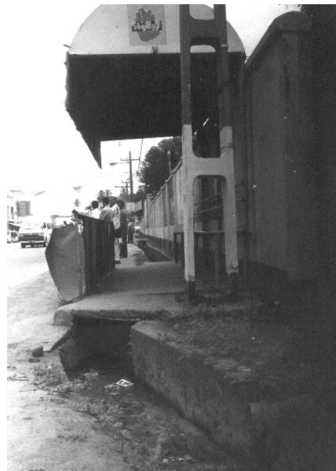
Figure 3.9 A bus-stand built over a drainage channel along Negombo Road, Kandana.
